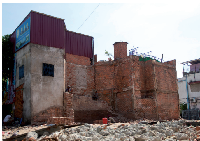
Demolished Ministry of Industry, Mines and Energy
